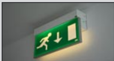
Measuring the emergency lighting in emergency exits
